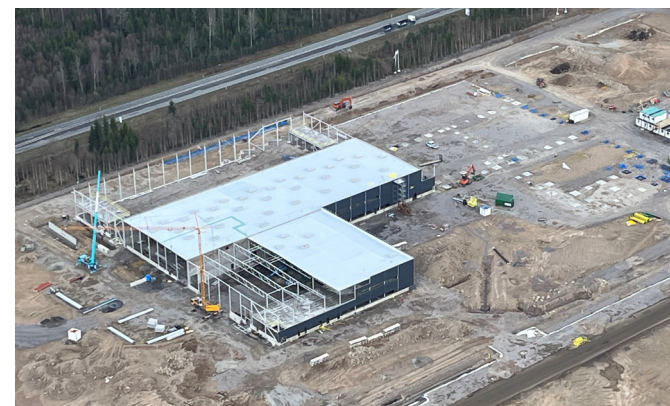
Phase 1 – Production for chargers. Picture from spring 2023.
